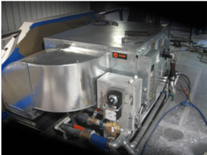
One of the air handlers, shown during installation on the Sky Deck
